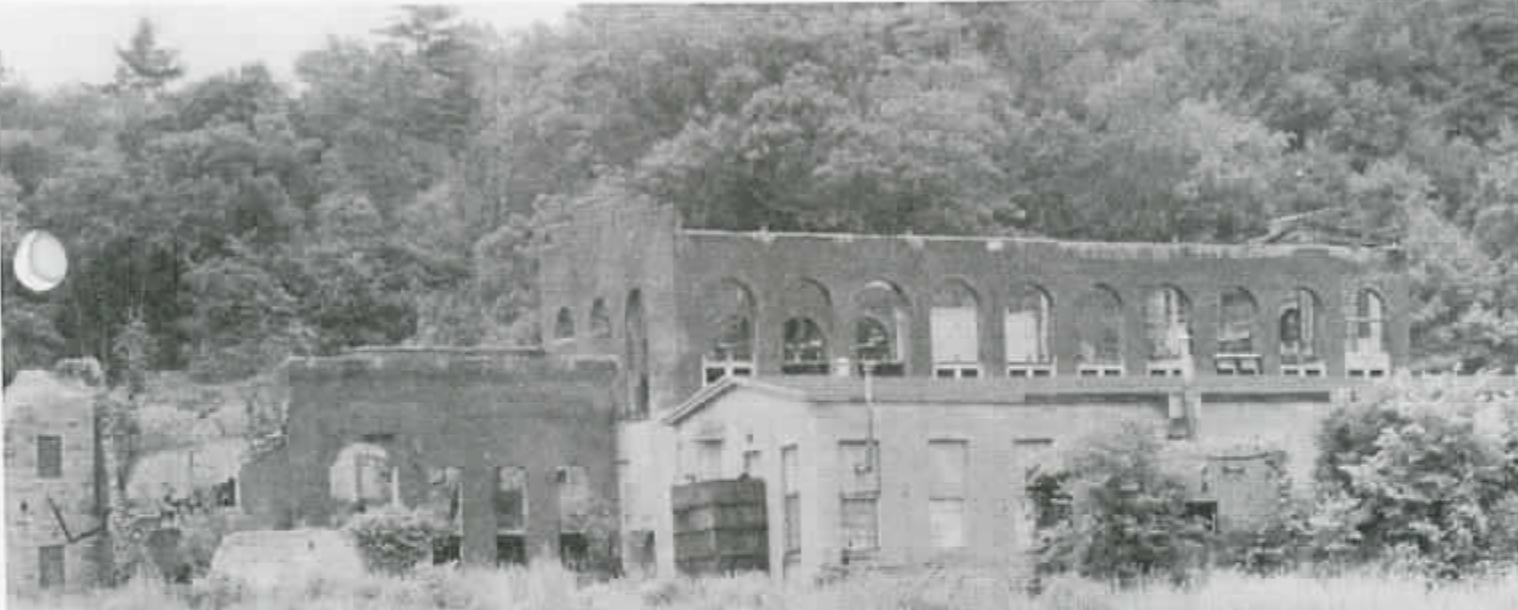
The "center" of the typical New England industrial town was the Mill, which often dominated the economy and even the politics of the town. The above ruin, photographed in far northeastern Connecticut in 1992, is just one example of what once was an extremely important part of the economy of New England.
